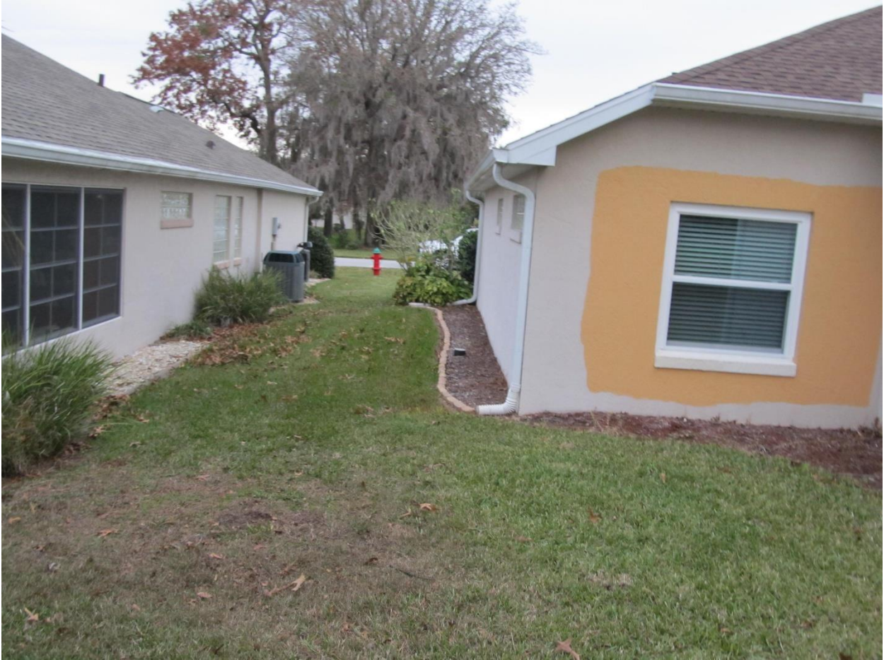
Looking at the westside of house from south property line.
