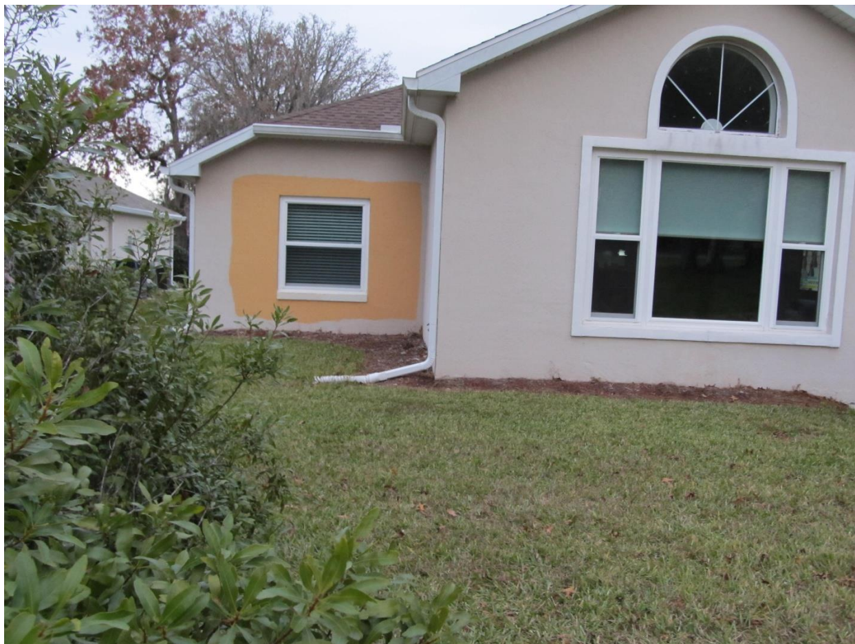
Looking north at rear of house from south property line.
