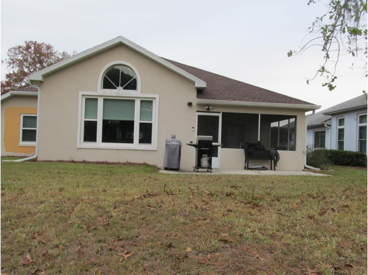
Looking at rear of house from south property line.
