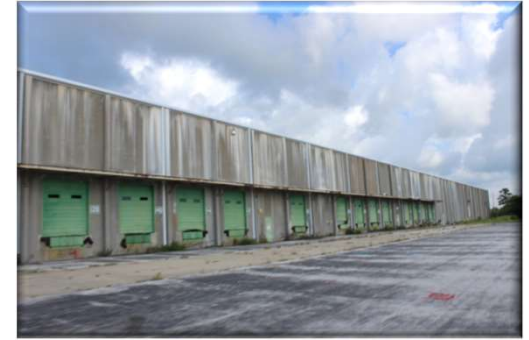
Rear Loading Area
