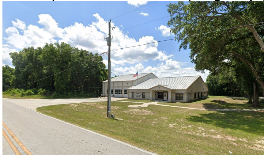
Figure 21. View of Spruce Creek Fire Station (Google Maps)
