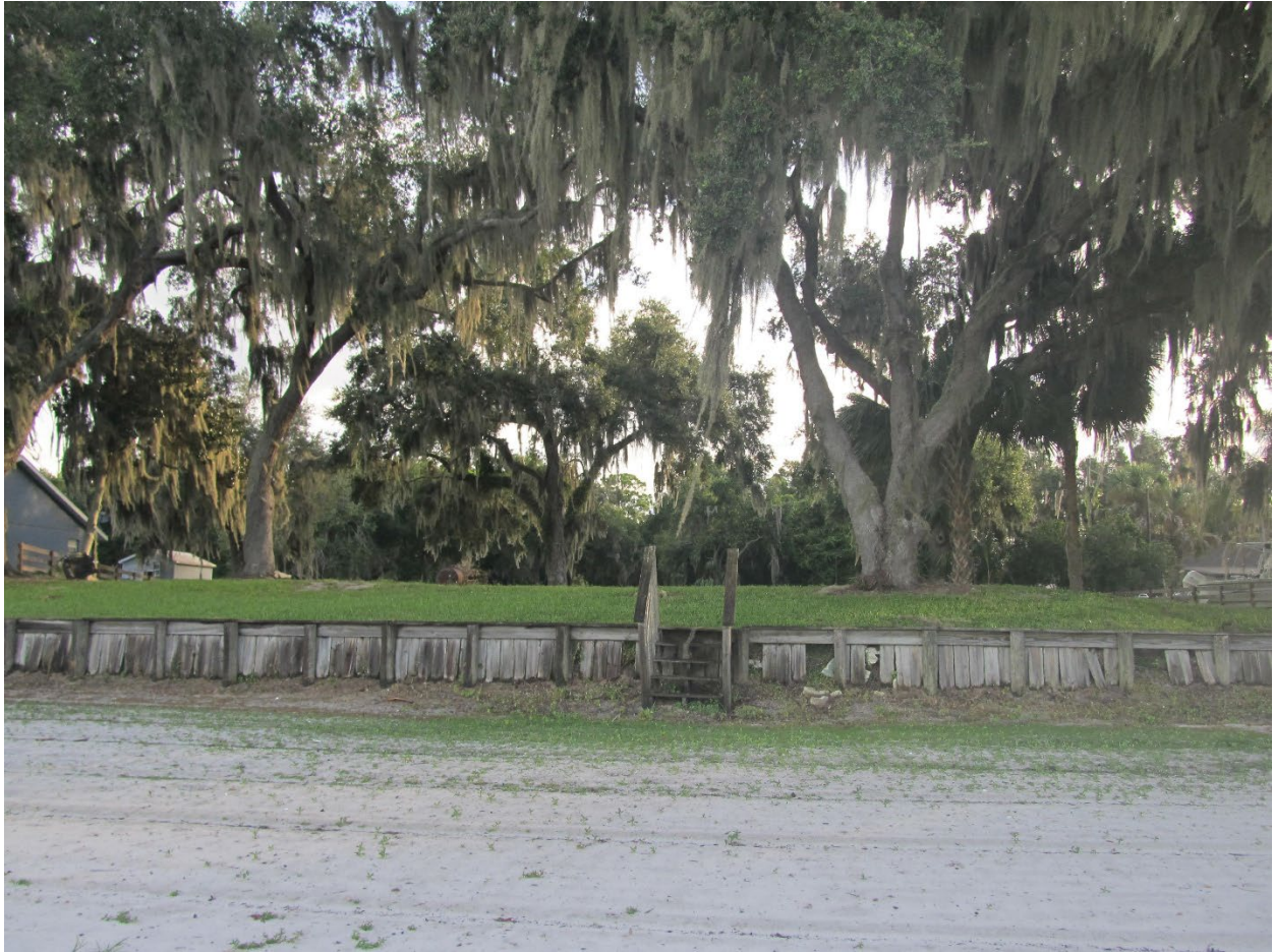
Looking north at seawall from waters edge.
