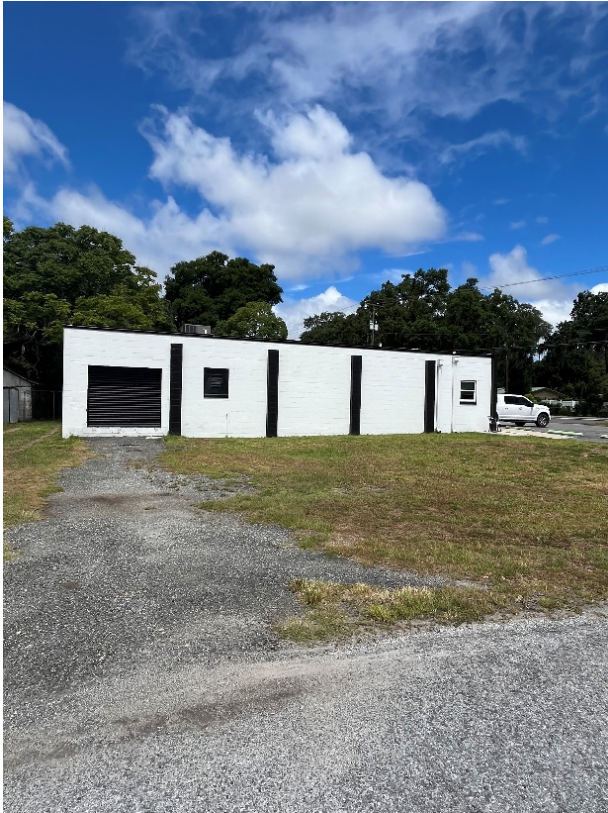
Side of existing building viewed from SE 134 th Ct.
