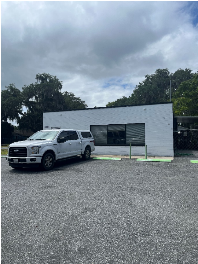
Existing building on subject site.
