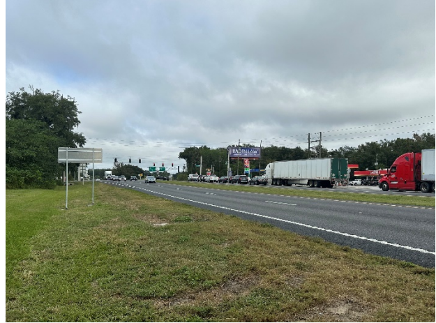
At subject property, along SB 441 looking north at the intersection of CR 329 and US Hwy 441.
