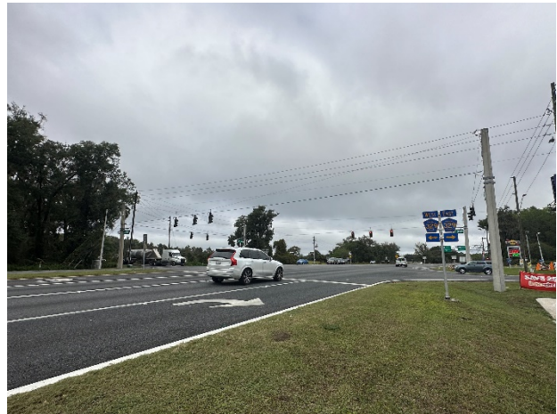
Circle K looking north at the NB side of the intersection of CR 329 and US Hwy 441.
