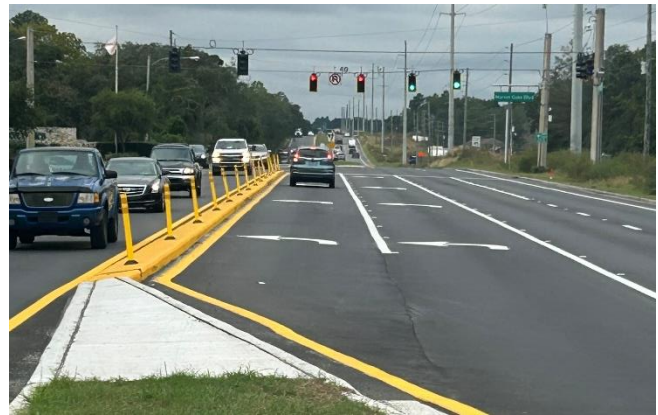
New westbound left turn lane on CR 484 at Marion Oaks Blvd
