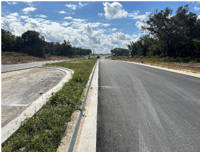
Newly paved section of SW 49th Ave Phase 1 just north of SW 66th
