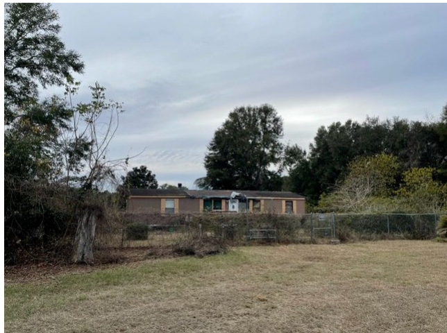
51. 1840 SW 130 th Street Road residence.
