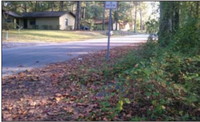
This photograph was taken from the West side of the road, at NE 56th Ave. No sidewalks, gutters, curbs, stormwater.
