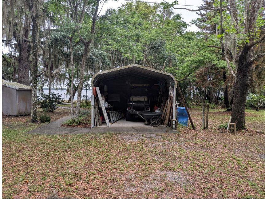
Figure 12. View of existing storage structure on PID 4938-001-000 (close-up)
