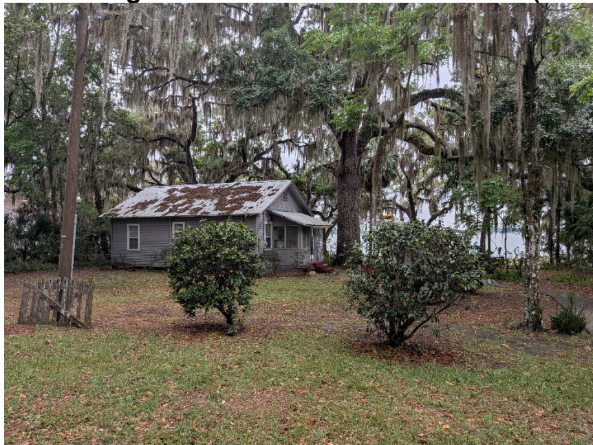
Figure 11. View of existing residence on PID 4938-001-000 (close-up)
