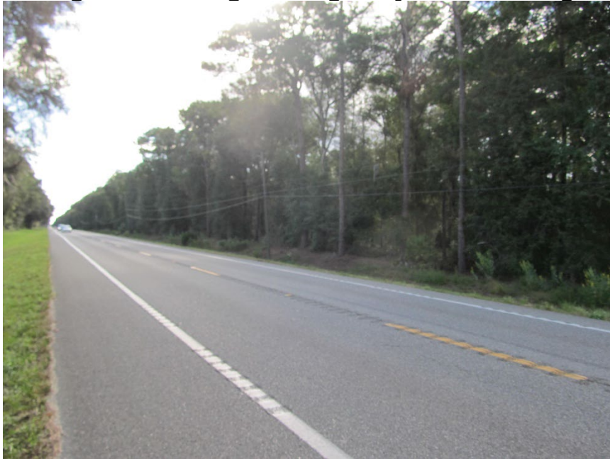
Figure 18. Facing south along SW Highway 200 from Sign D
