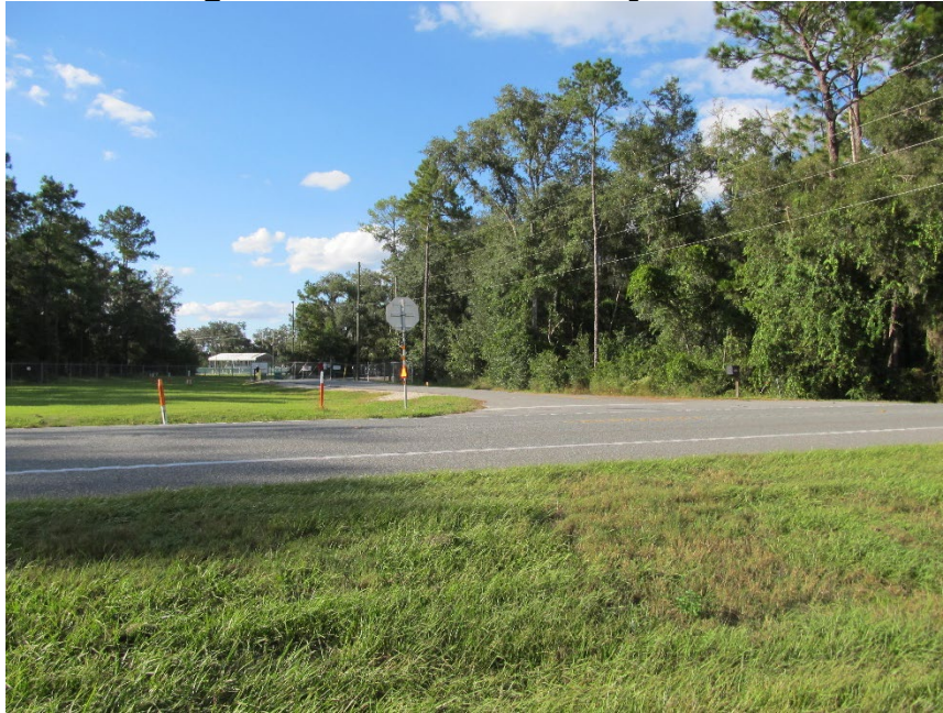
Figure 22. View of natural gas distribution facility on PID 40867-001-00
