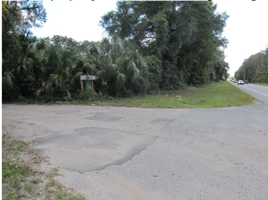
Figure 6. View of subject property main entrance along SW Highway 200
