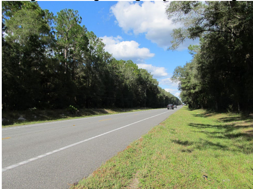
Figure 7. Facing north along SW Highway 200 from Sign B
