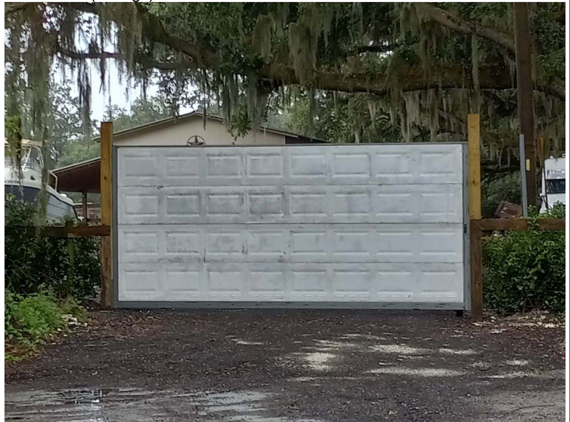
Exterior of Gate (Converted Garage Door)
