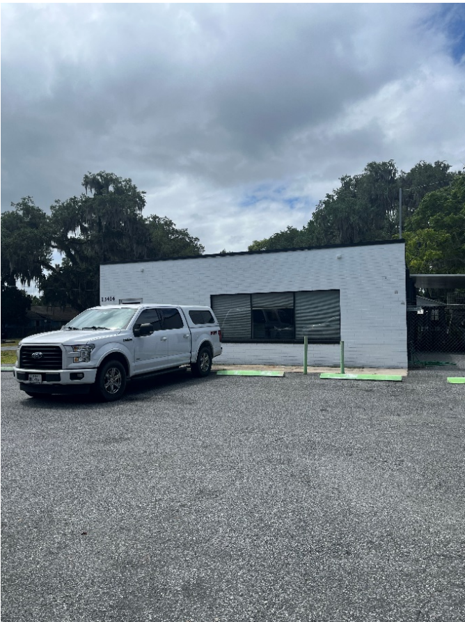
Existing building on subject site.
