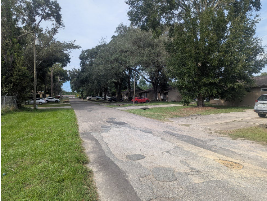
Figure 10. View of existing duplexes along NW 58 th Court
