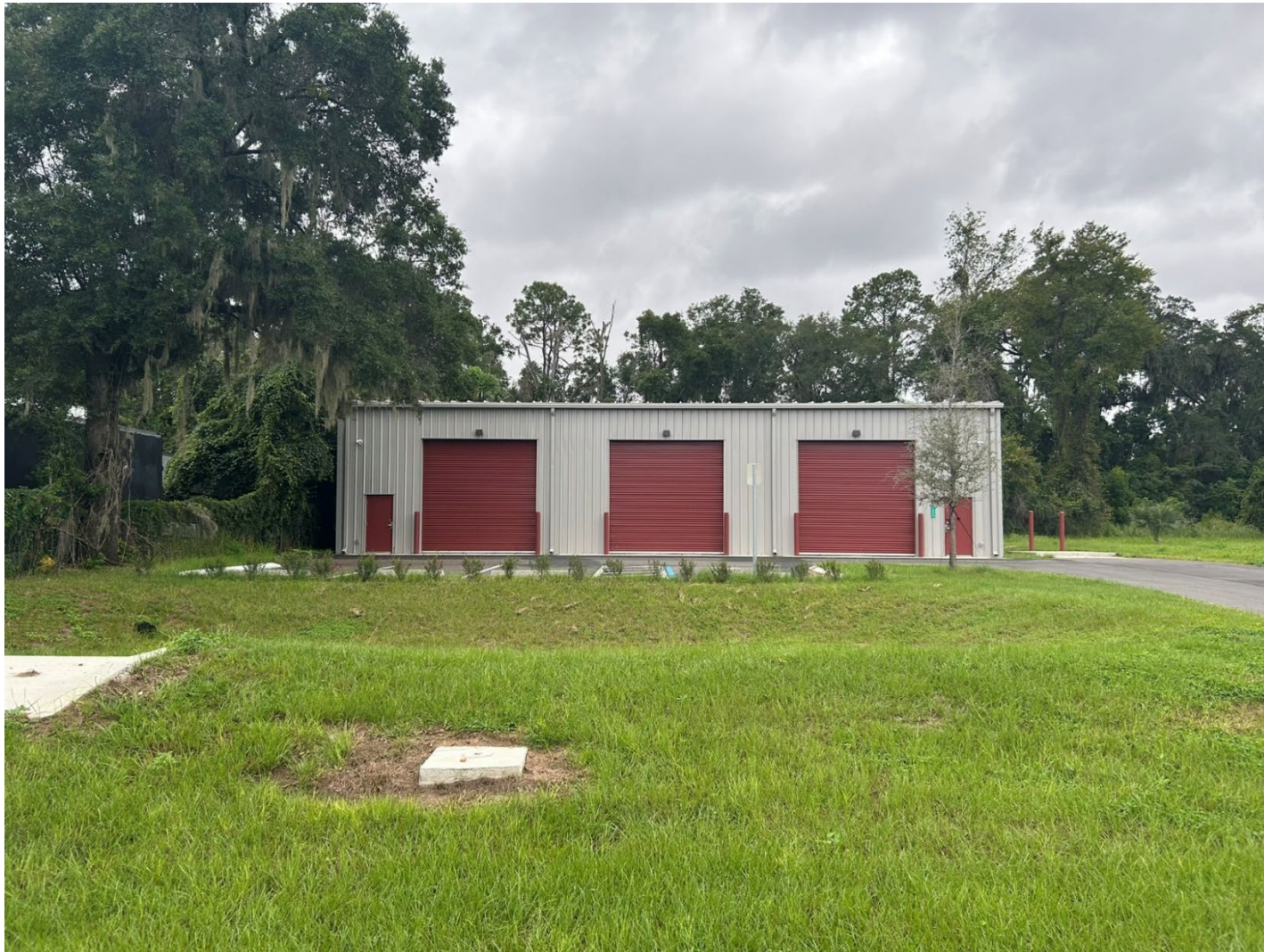
Figure 1 – Storage Warehouse, Front of Building, Facing S
