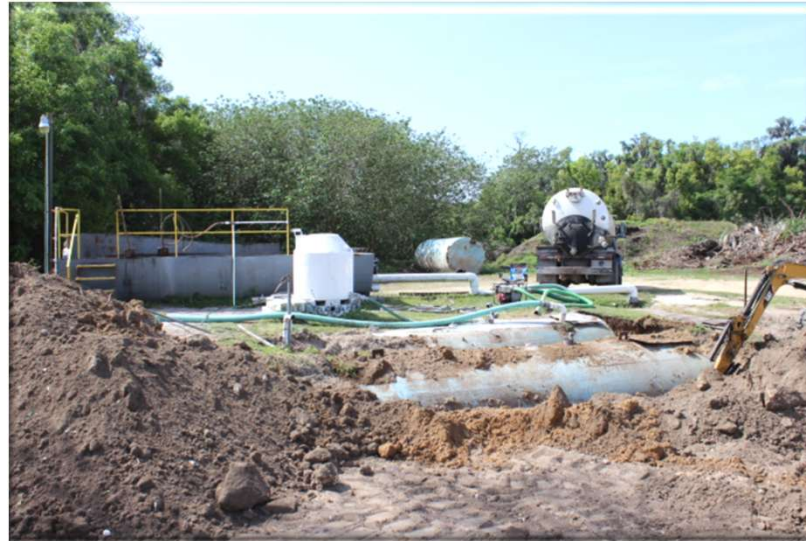
Septage System Removal
