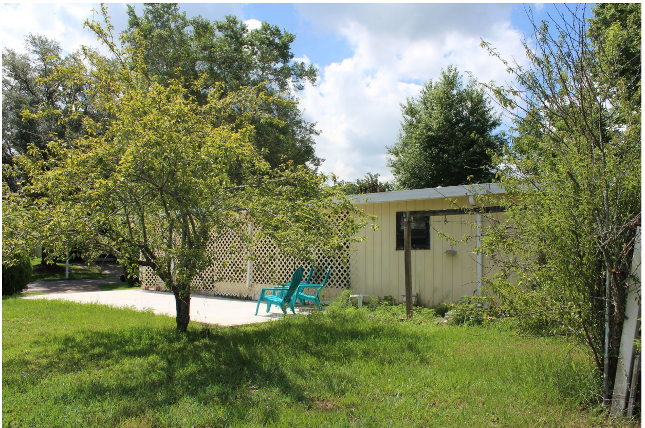
New concrete slab and existing carport with storage looking Southeast
