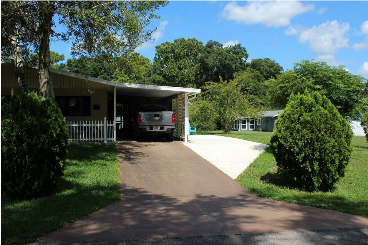
Facing West looking at the house and new slab
