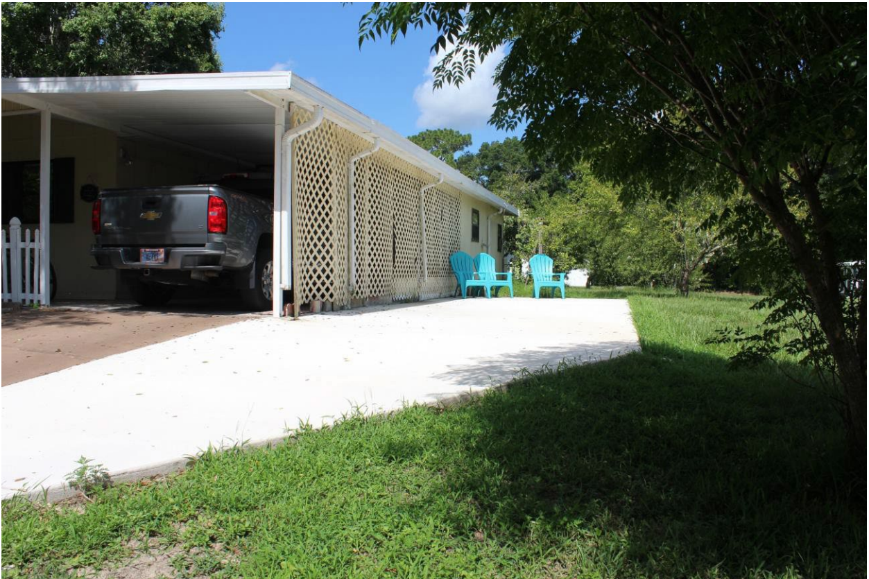
Close up of concrete slab looking west
