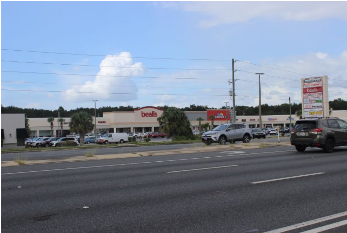
Looking across SW Hwy 200 to Steeplechase Plaza.
