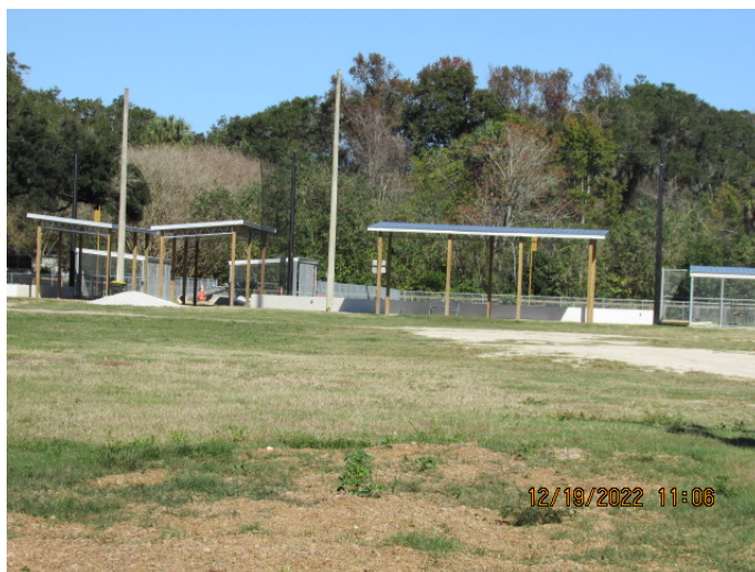
Photo of dugouts, fields, and stadium light poles.
