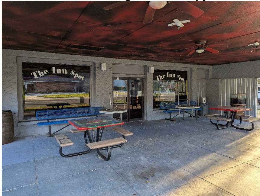
Figure 9. View of outdoor seating under canopy structure
