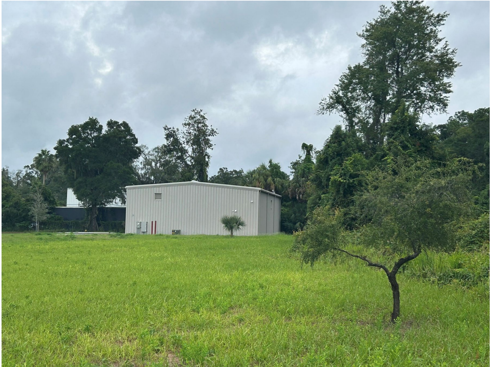
Figure 2 –Storage Warehouse, Side and Rear of Building, Facing NE
