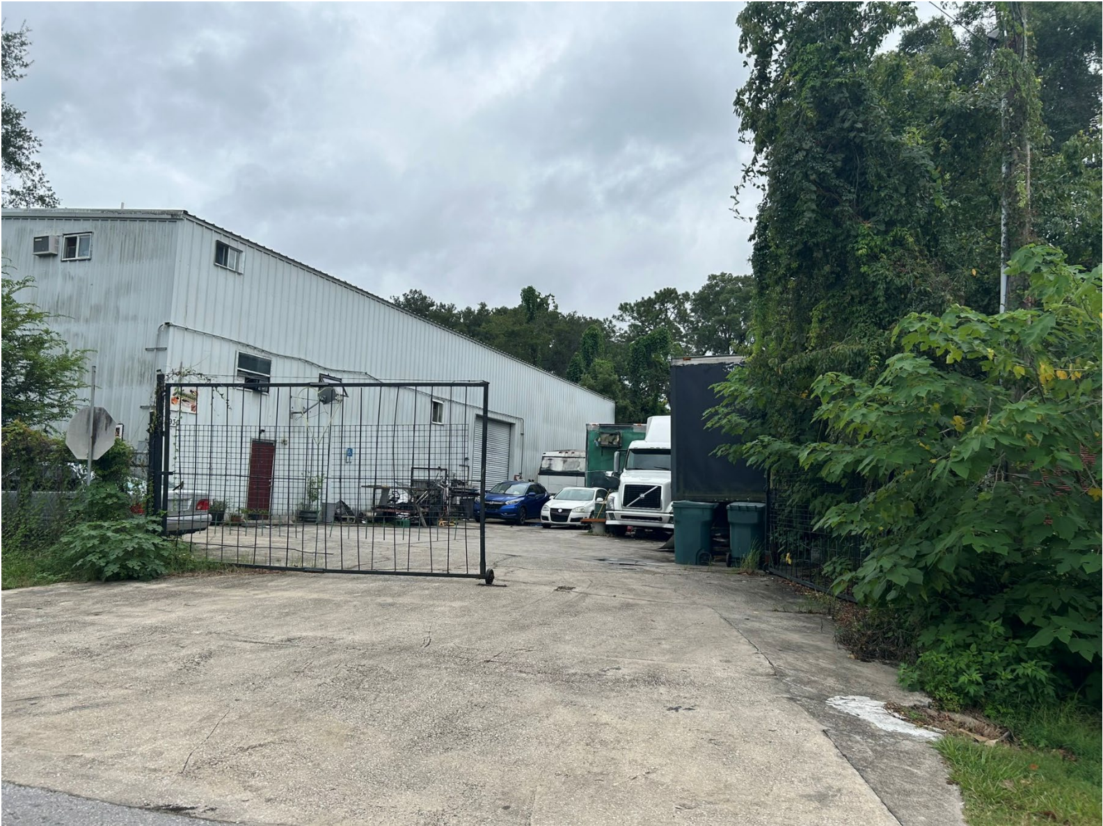
Figure 6 – E Neighboring Property, Facing S, along 1920-30 BLK of NE 20 th Street
