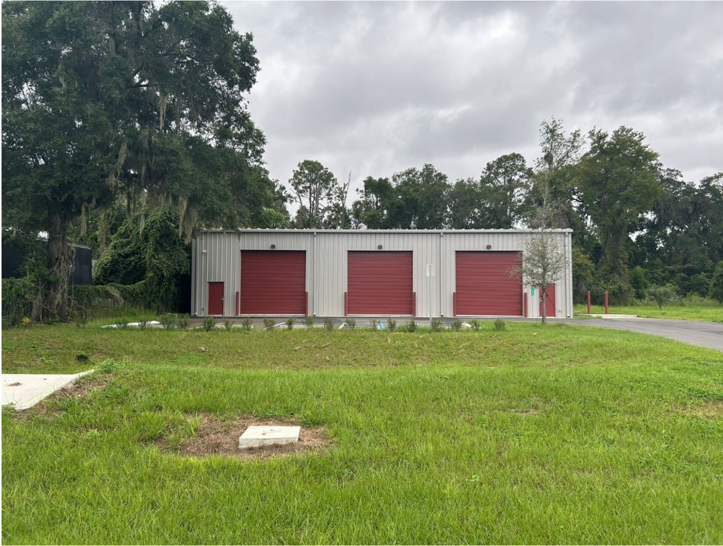
Figure 1 – Storage Warehouse, Front of Building, Facing S
