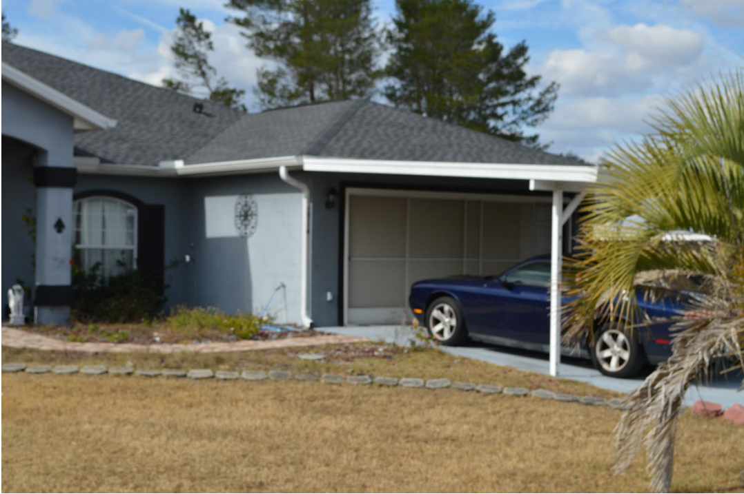
Looking at southside of carport
