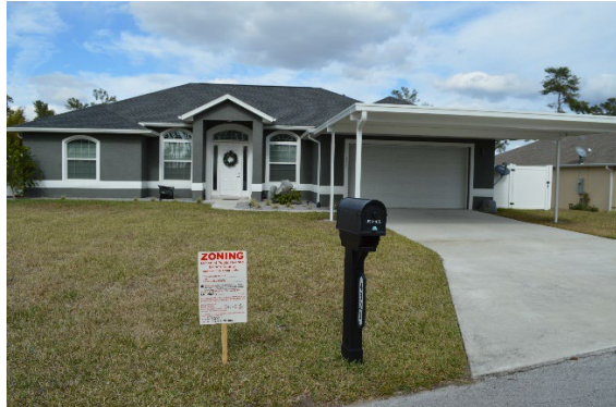
Figure 3 House with subject carport
