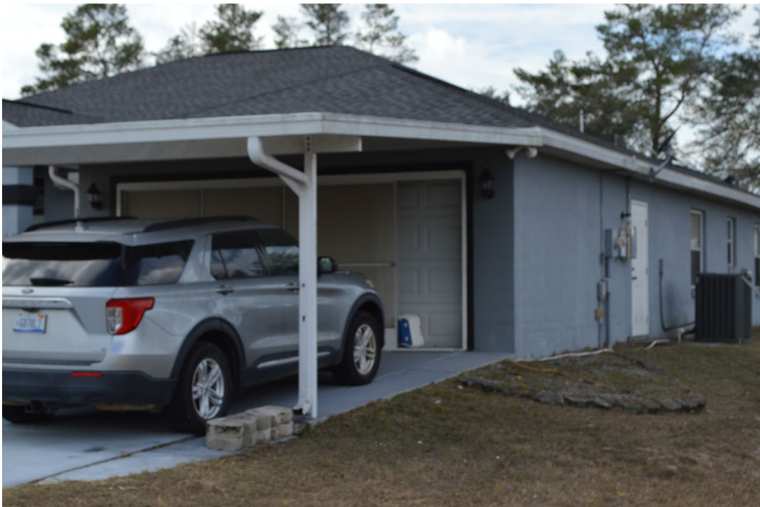
North side of carport
