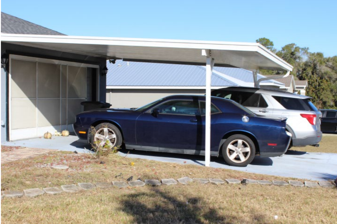
South side of carport
