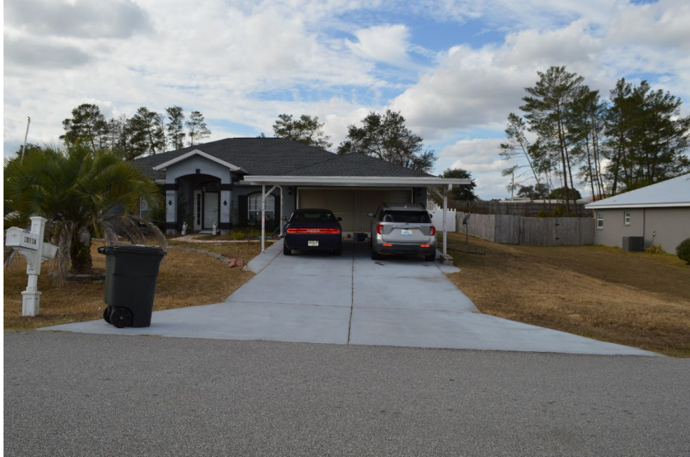
Looking west towards carport
