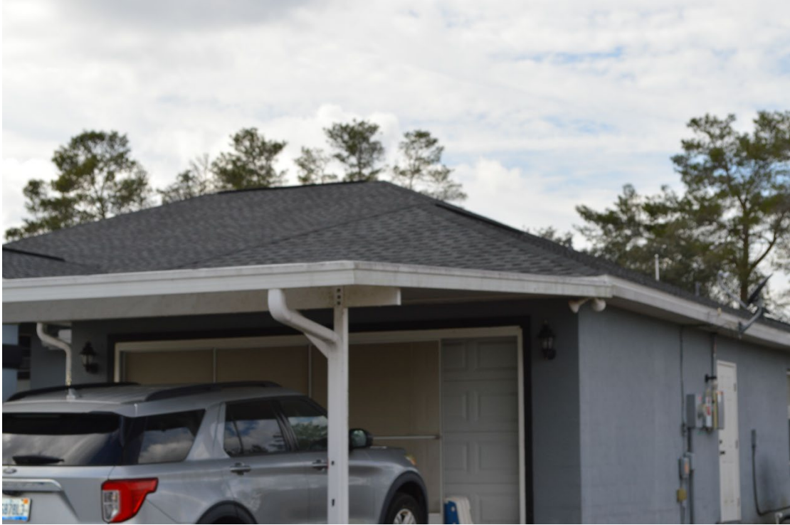
North side of carport
