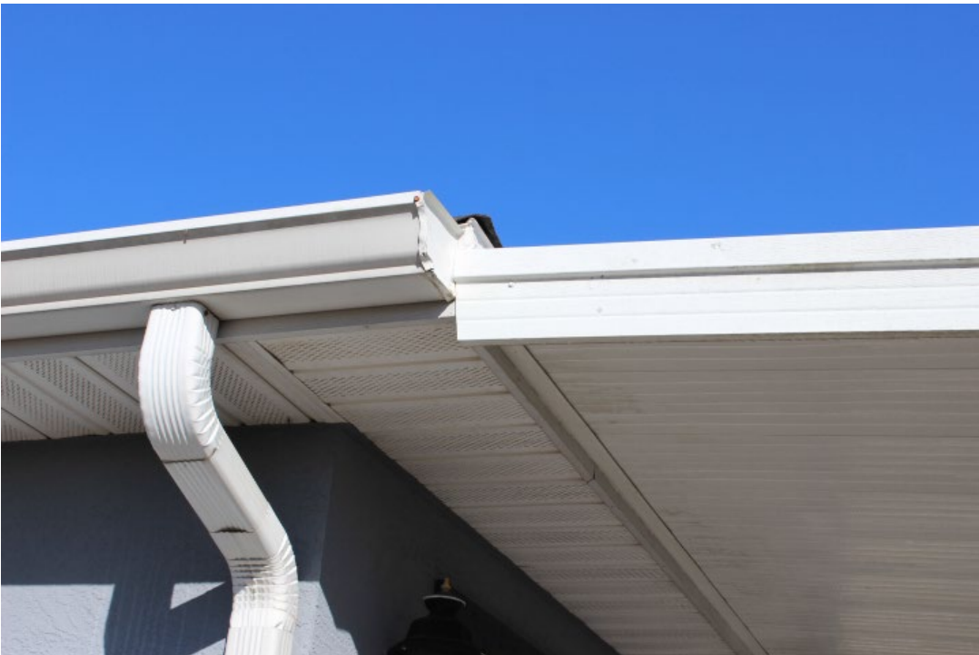
Southside of carport roof connection
