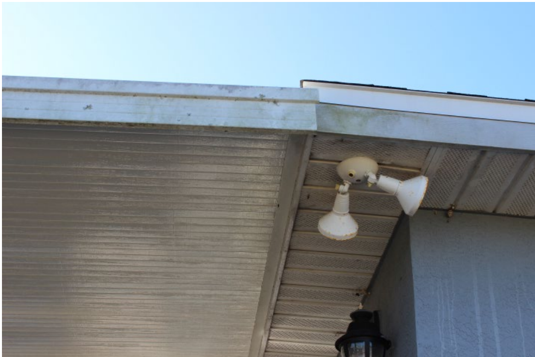
North side of carport roof connection
