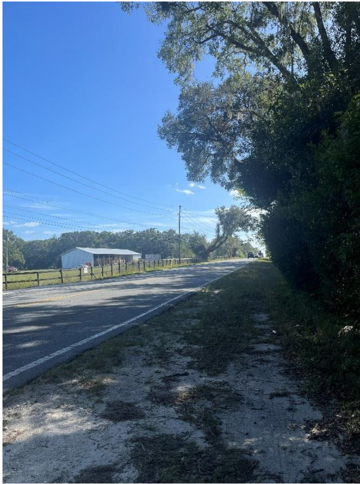
Looking south on NW Gainesville Road.
