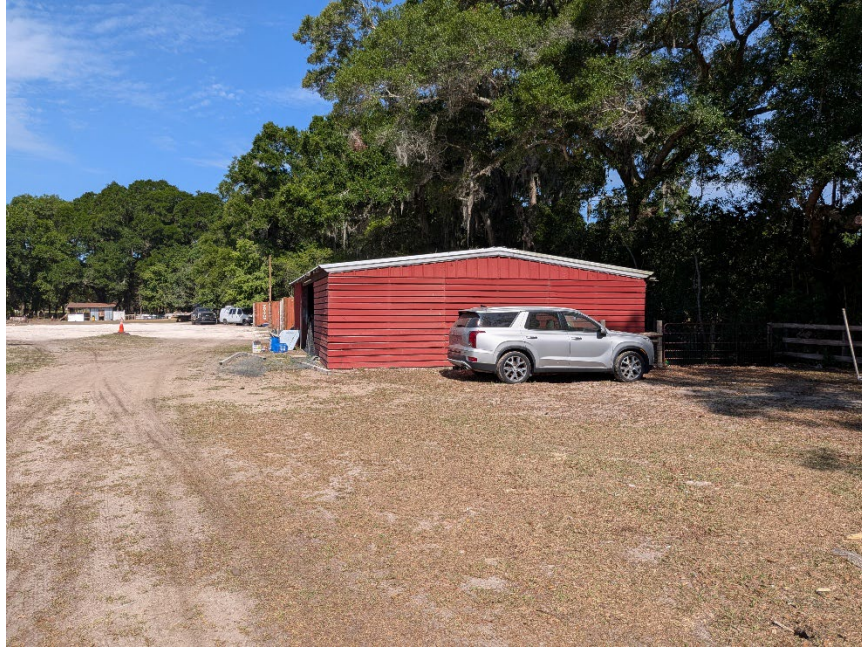
Figure 10. View of accessory structure along northern subject property boundary
