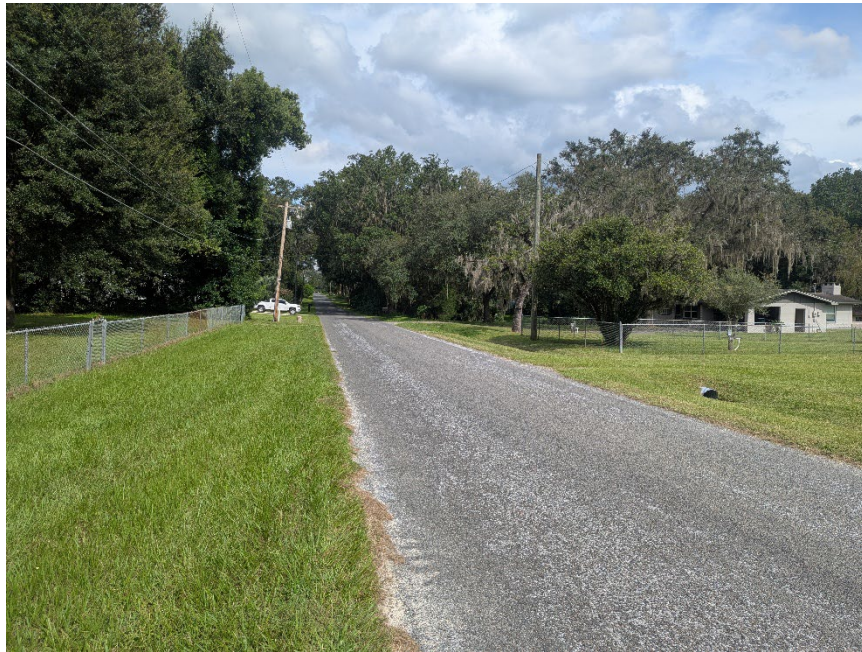
Figure 20. View of SW 73 rd Street Road in Hamblen H.A. subdivision
