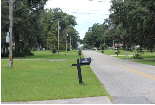
Figure 7 facing east from driveway
