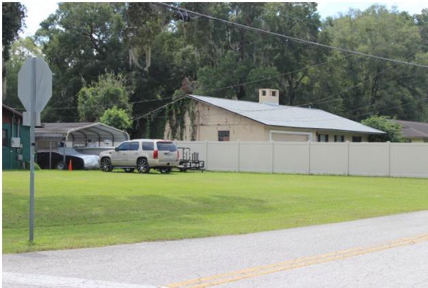
Figure 13 facing southwest across subject property
