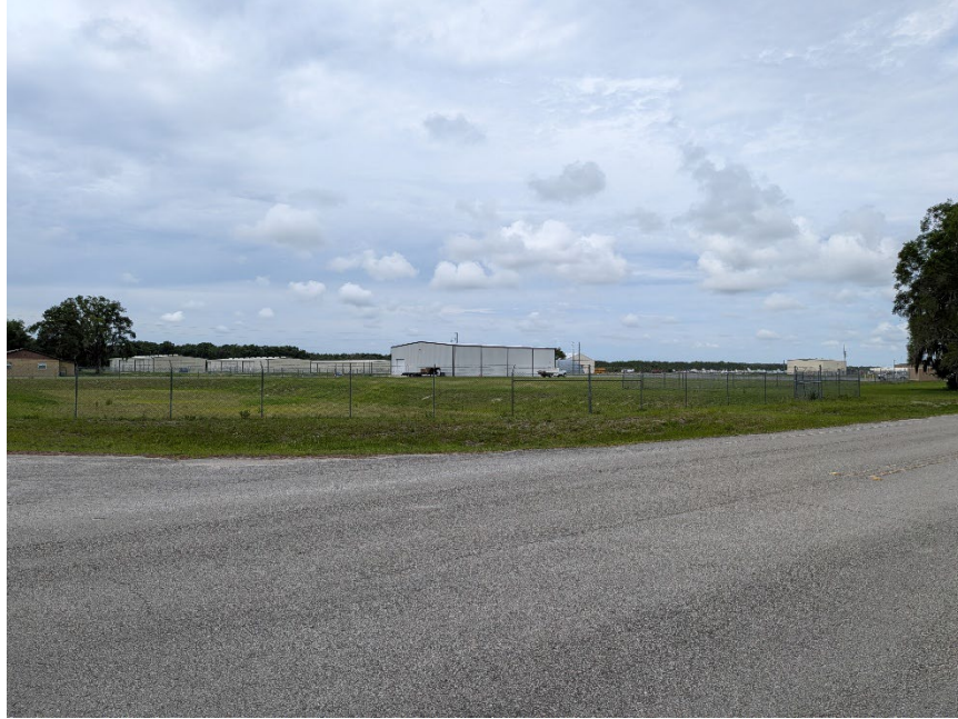
Figure 20. View of hanger buildings adjacent to Marion County Airport terminal
