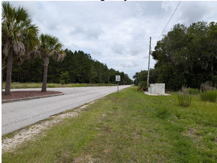
Figure 15. View of SW 147 th Court from Marion County Airport entrance along SW Highway 484
