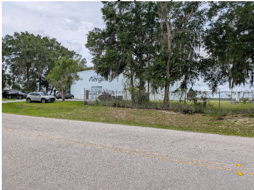
Figure 22. View of aviation-related industrial buildings adjacent to existing taxiways (cont...)
