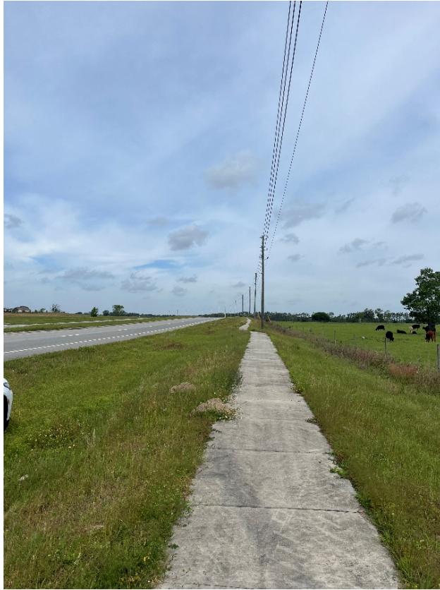
Looking north on SE 92 nd Loop
