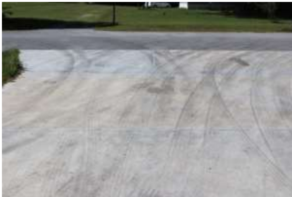
Improved driveway on SW 15 th Place
