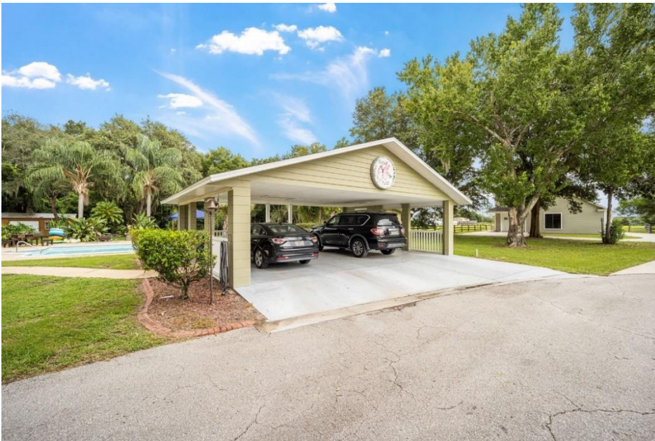
A view of the parking deck.
