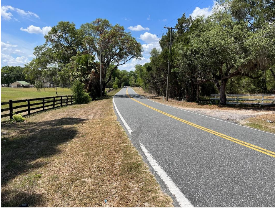
On SE 110 TH Street Road facing west.
