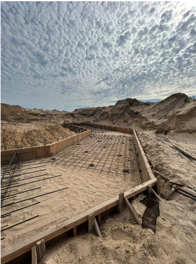
Emerald Rd Extension – Cattle Tunnel Footer Construction
