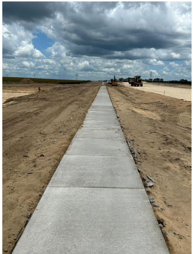
Emerald Rd Extension – Sidewalk Installation
