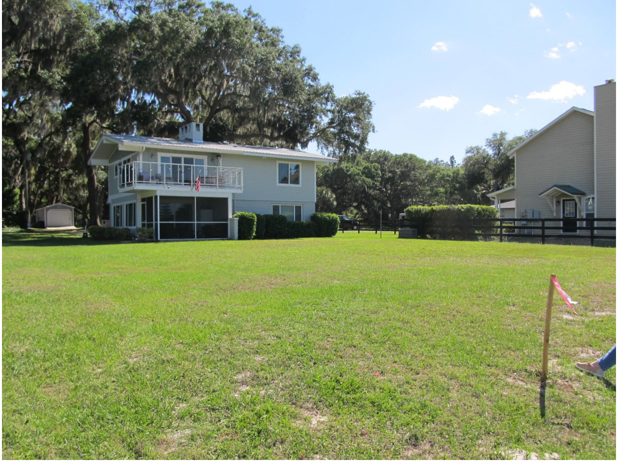
Looking southwest at the proposed pool with deck area
