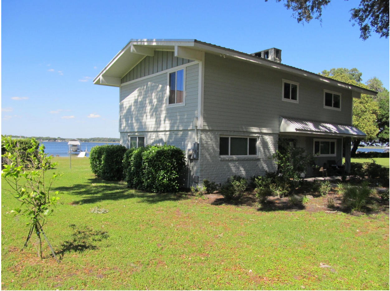
Looking northeast at home (side yard)
