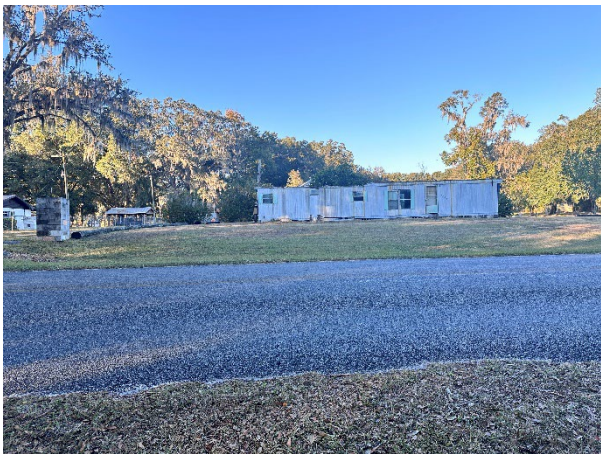
Property across SE 62 St
