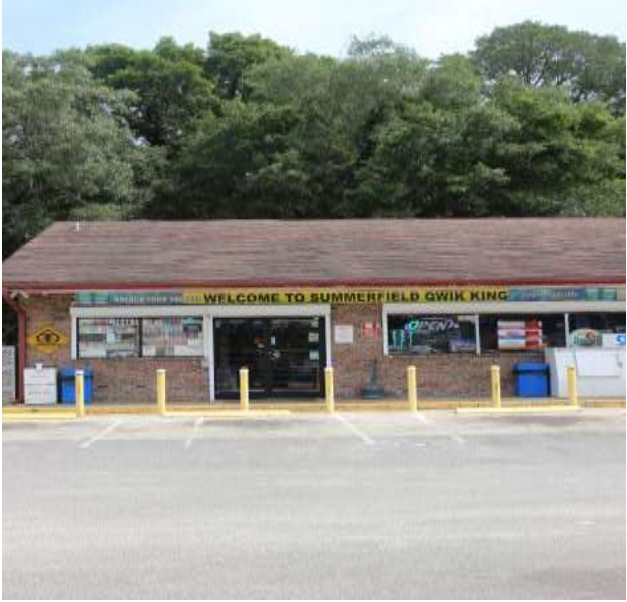
Retail Store (Eligible Under Policy 1.20 Letter) on subject parcel, located at intersection of HWY 42 and HWY 301
