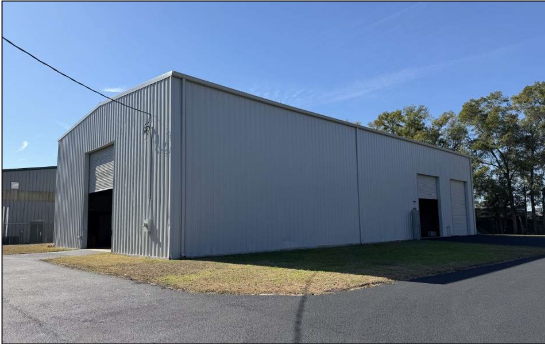
Close-up front view of the warehouse building at the rear of the site.
