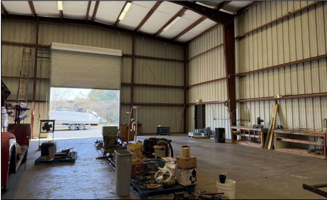
Current interior view of the warehouse building on the site.
