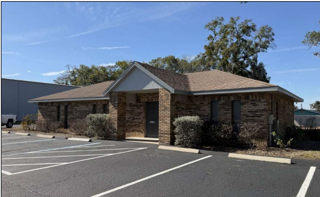
Close-up front view of the office building at the front of the property.
