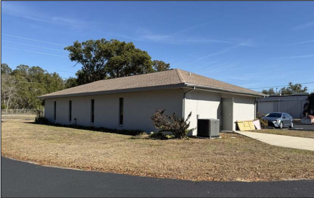
Close-up rear view of the office building at the front of the site.
