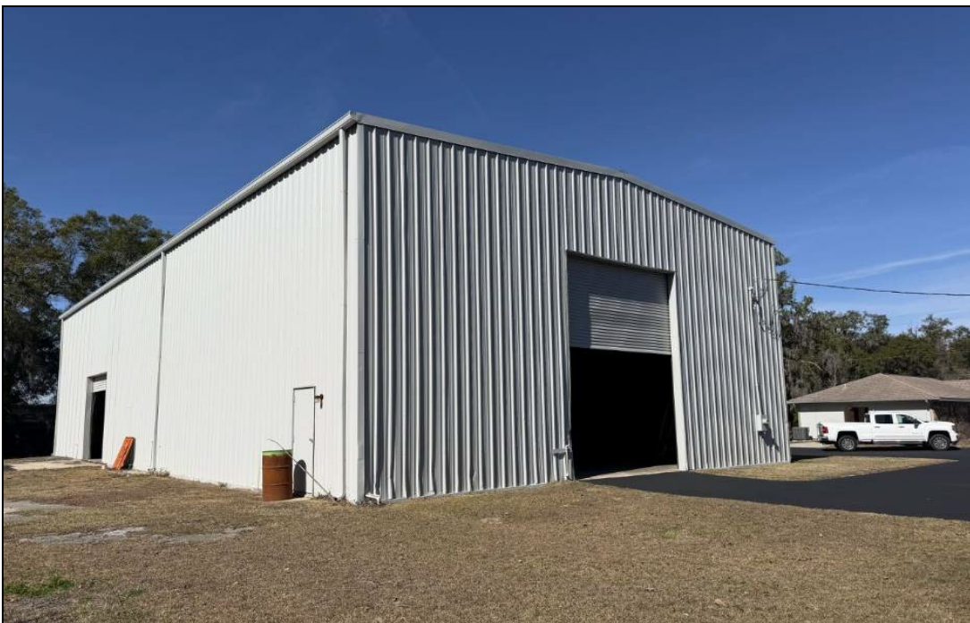
Close-up rear view of the warehouse building.
