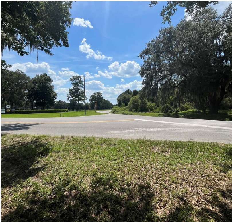
Intersection of NW 110 th Ave. and NW Hwy 464B.
