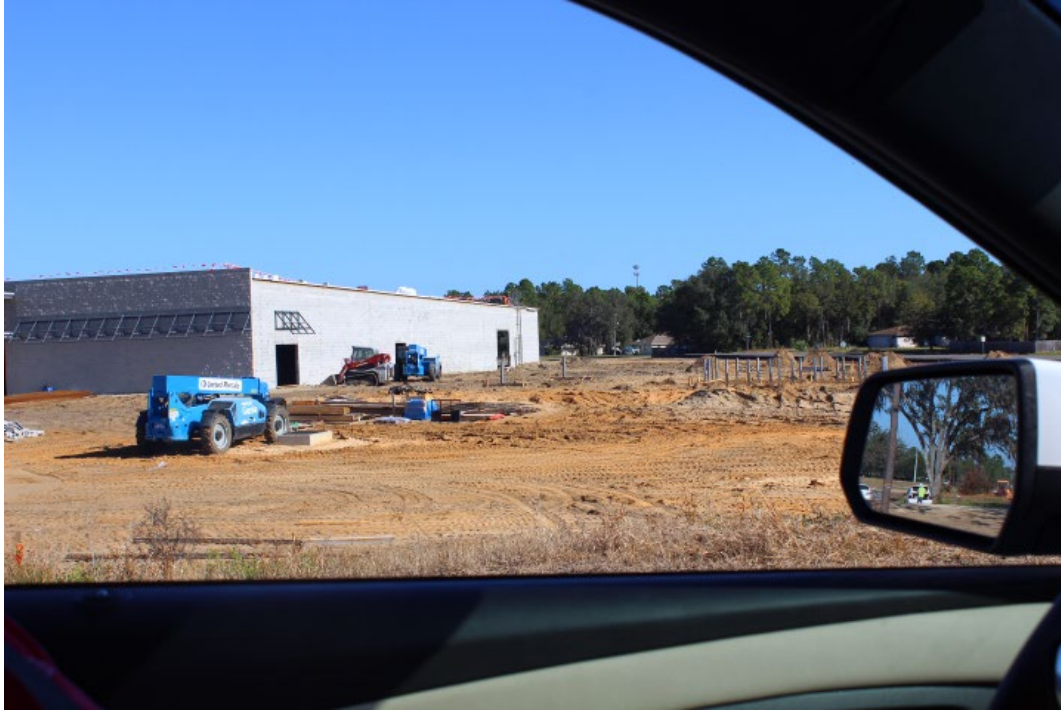
Looking West at the rear of the structure.
