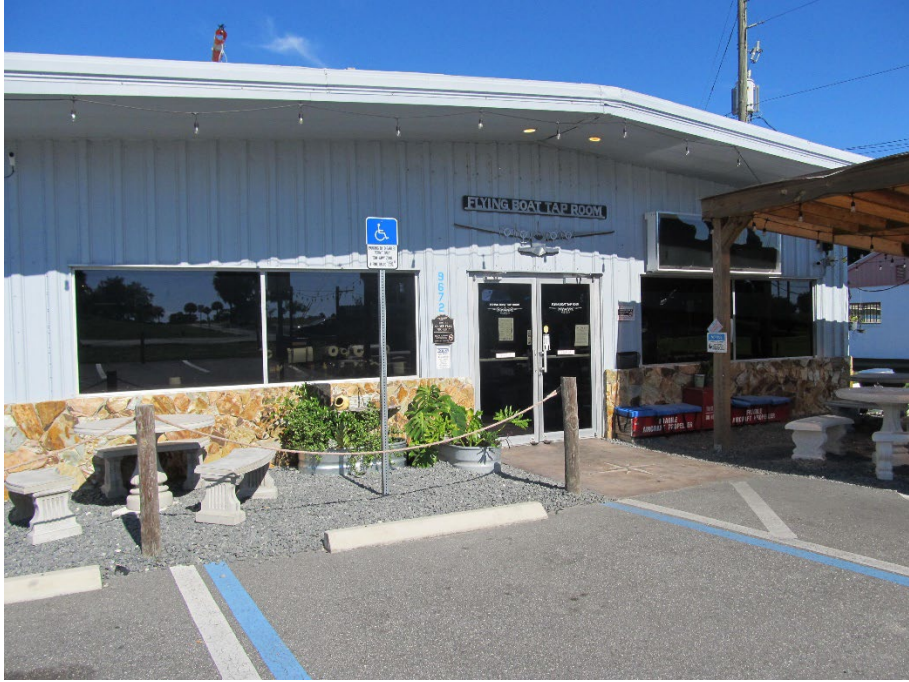
Front of main structure with address on the front
