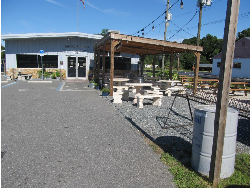
East (Front) looking West at the front of the building. Pergola on right
