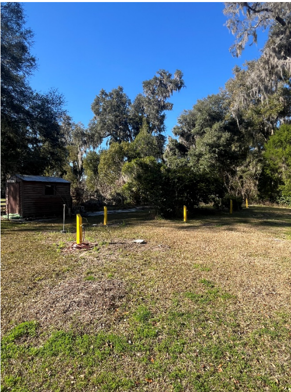
Close up of RV hook-ups (Shed shown in background).
