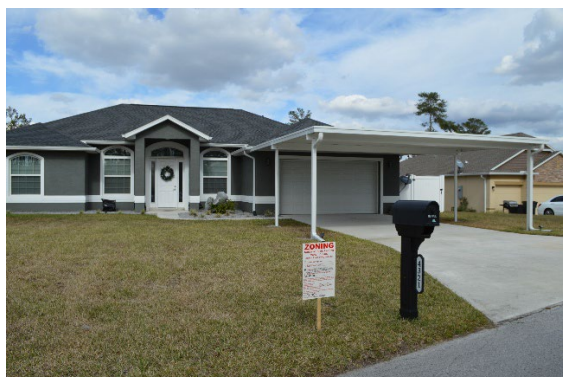
Figure 5 Subject carport showing attachment to building
