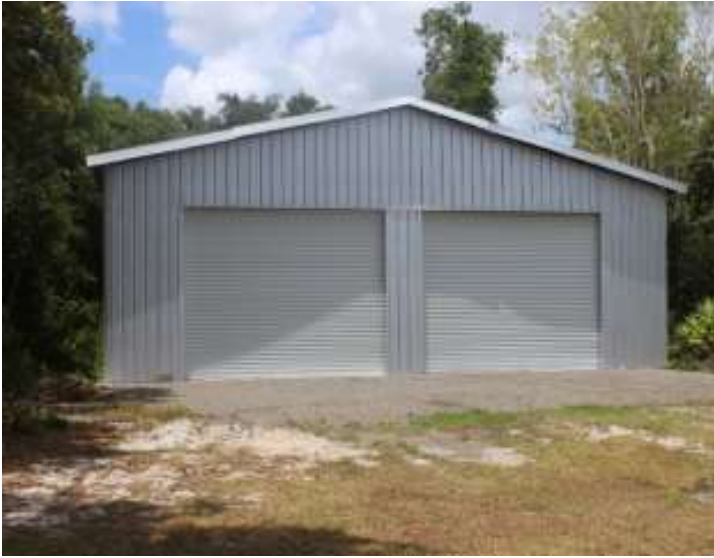
Front view of the structure, located on NE 243 rd CT
