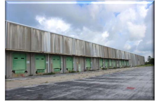
Rear Loading Area
