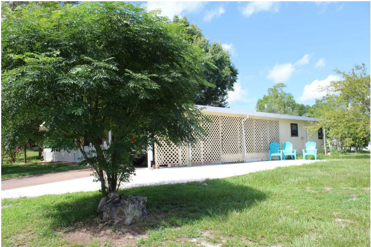
Entire existing carport and storage with slab looking Southwest
