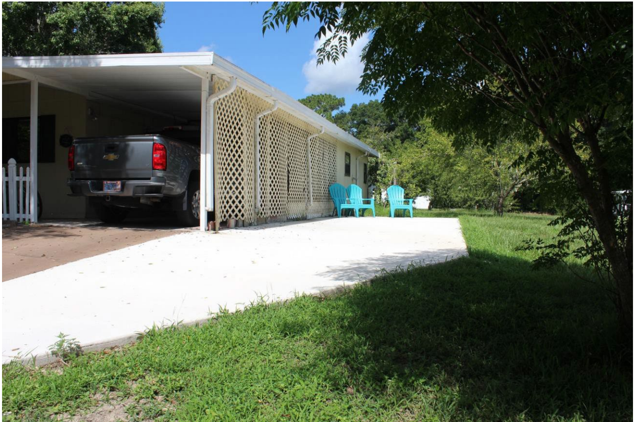
Close up of concrete slab looking west
