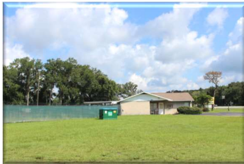
South Side of Primary Bldg
