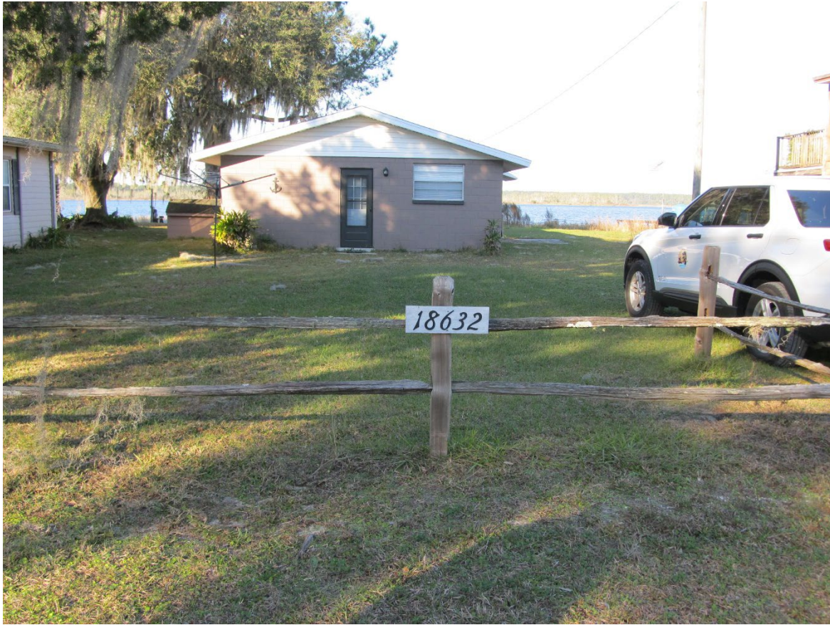
Looking at the front of the property with the address.
