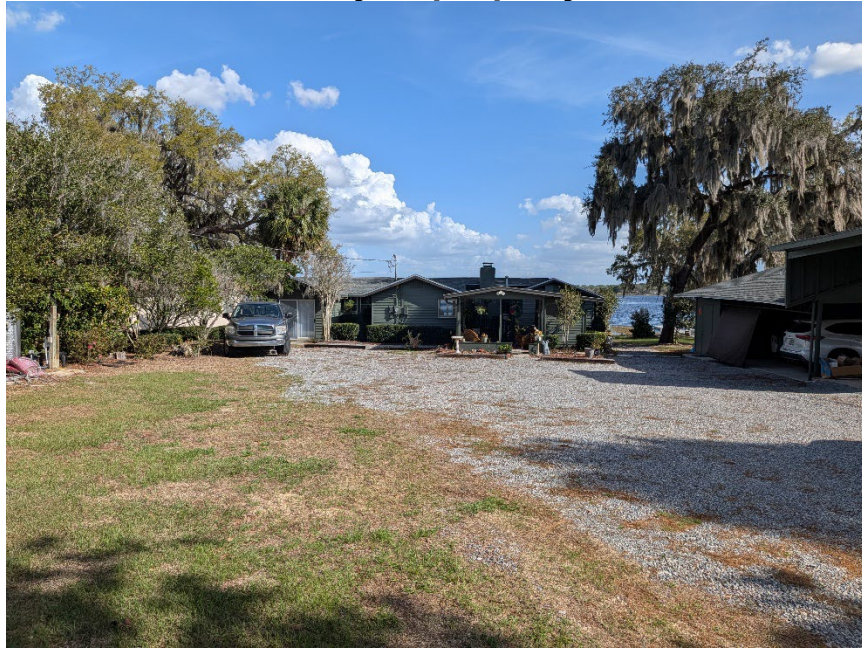
Figure 4. Facing south toward front of existing single-family residence on subject property
