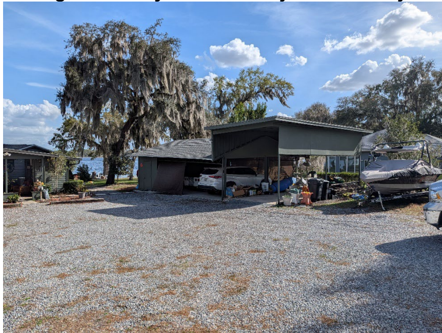
Figure 5. View of existing accessory structure adjacent to subject residence
