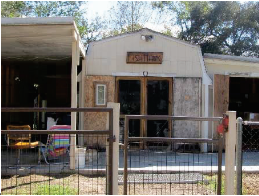
3. View of distillery building.
