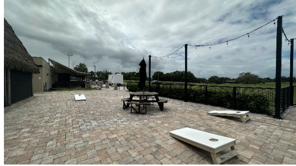
Existing gaming facility (outdoor space). Without permit.
