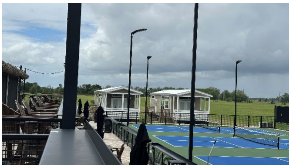
Existing gaming facility (outdoor space), pickleball courts, manufactured buildings. Without permit.
