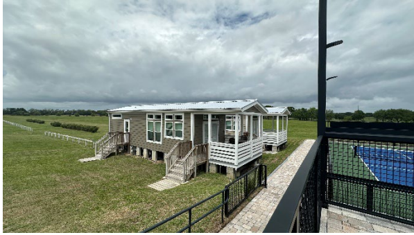
Existing manufactured trailers/buildings (office and storage use). Non-conforming use, without permit.
