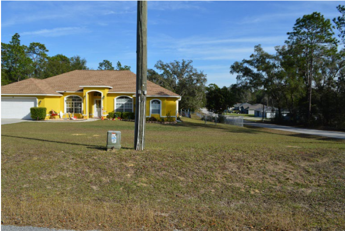
Residence across the street on SW 204 th Ave.
