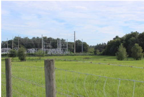
Figure 10 facing north towards SECO substation
