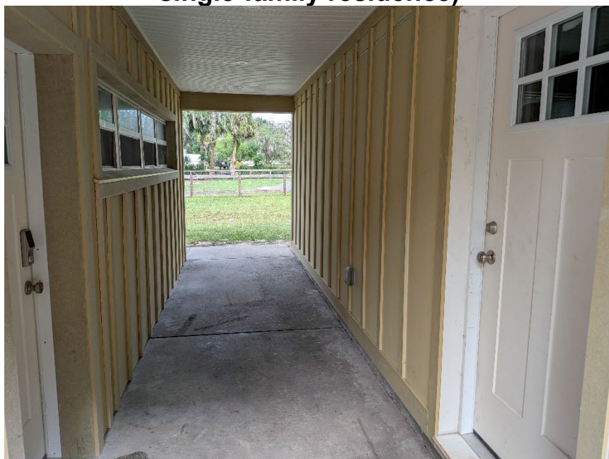
Figure 10. View of outdoor corridor between garage and kids room (part of single-family residence)
