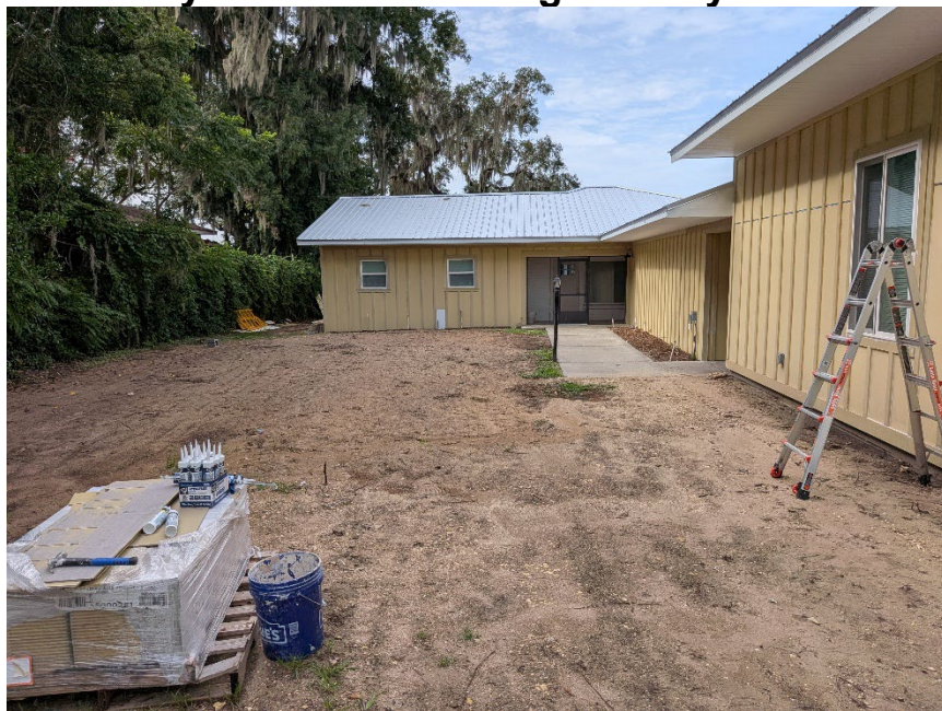
Figure 12. View of yard in front of single-family residence
