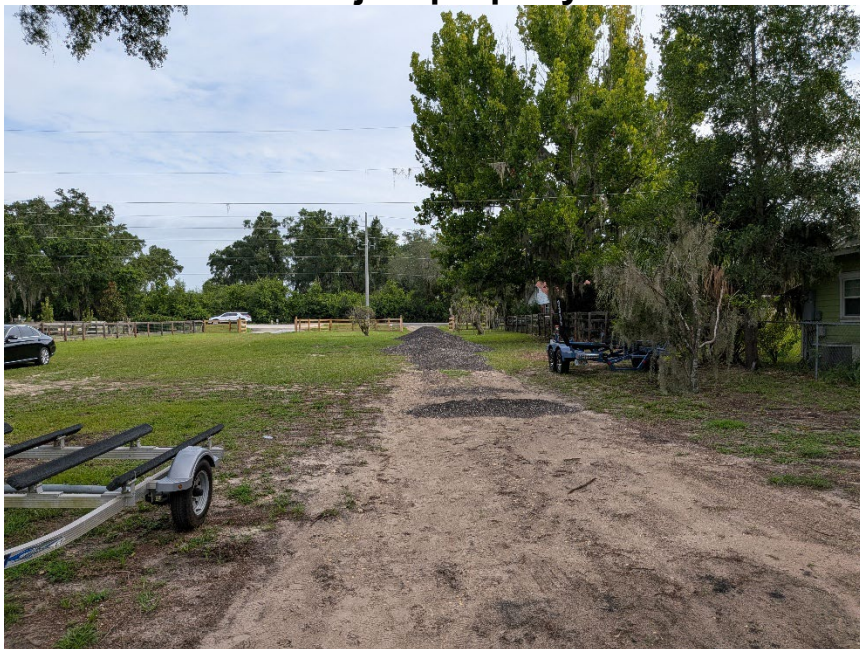
Figure 5. View of driveway (in progress) leading to single-family residence on subject property
