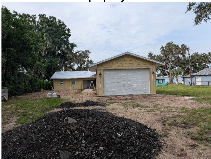
Figure 7. View of garage and single-family residence (in progress) on subject property
